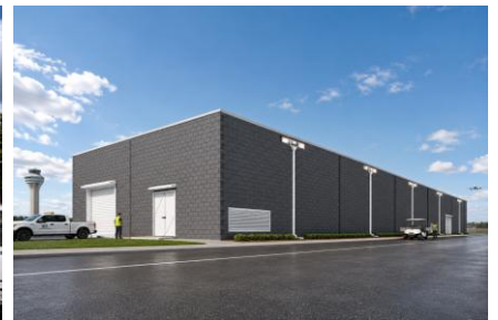
Hartsfield-Jackson S. Airfield Lighting Vault Bldg Government + Civic | Atlanta, Georgia
